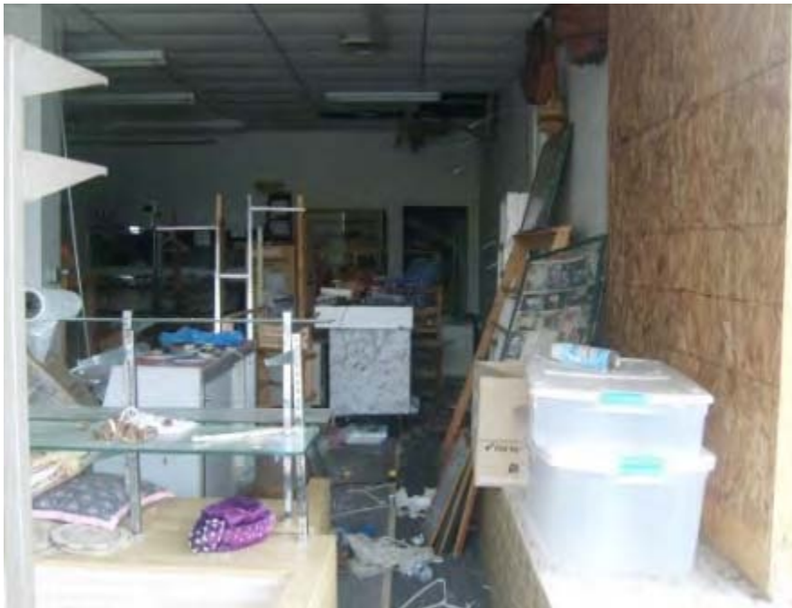
Photo No. 6: View of interior.
