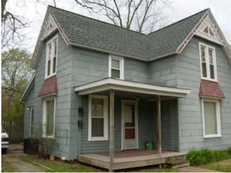
Photo No. 7: View of northerly adjacent residential property (9 Ballard Street).
