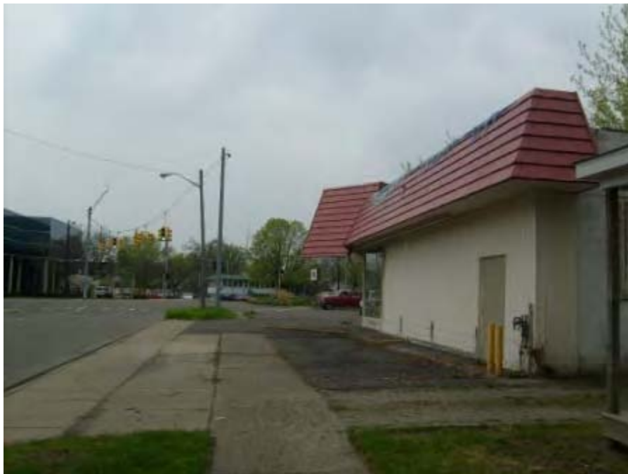
Photo No. 2: Looking south at the east boundary of the site from near the northeast corner of the site.
