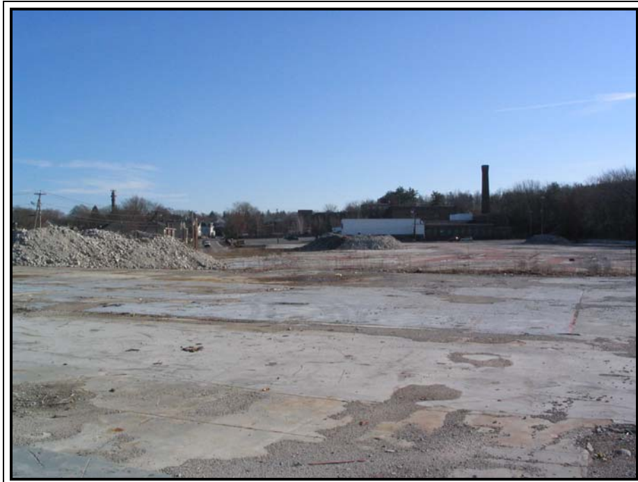
View of 172 Sterling Facing Southeast
