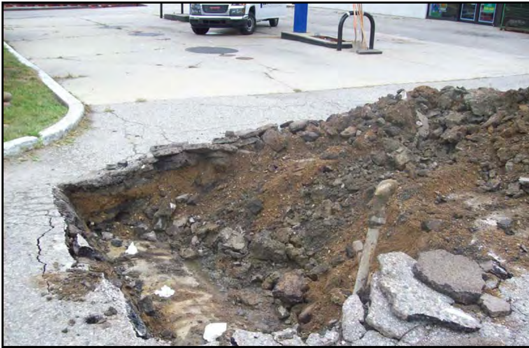
PHOTOGRAPH 7: 550-GALLON UST WITHIN TEST PIT #2
