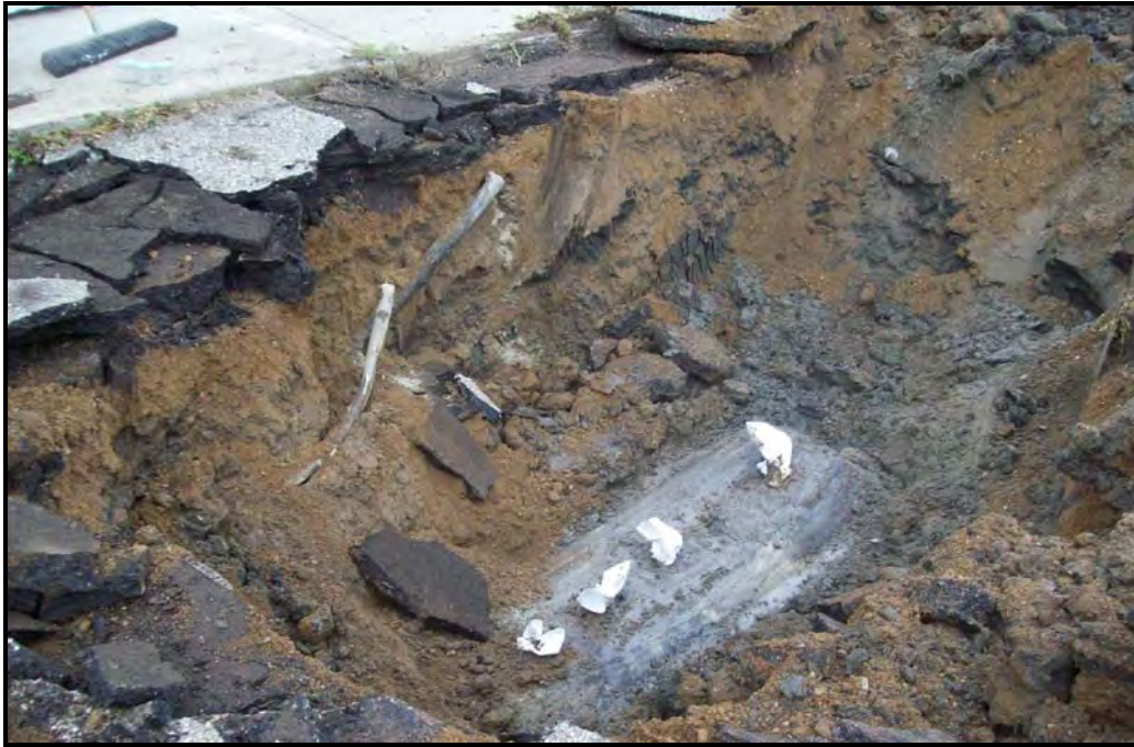
PHOTOGRAPH 3: 550-GALLON UST WITHIN TEST PIT #1
