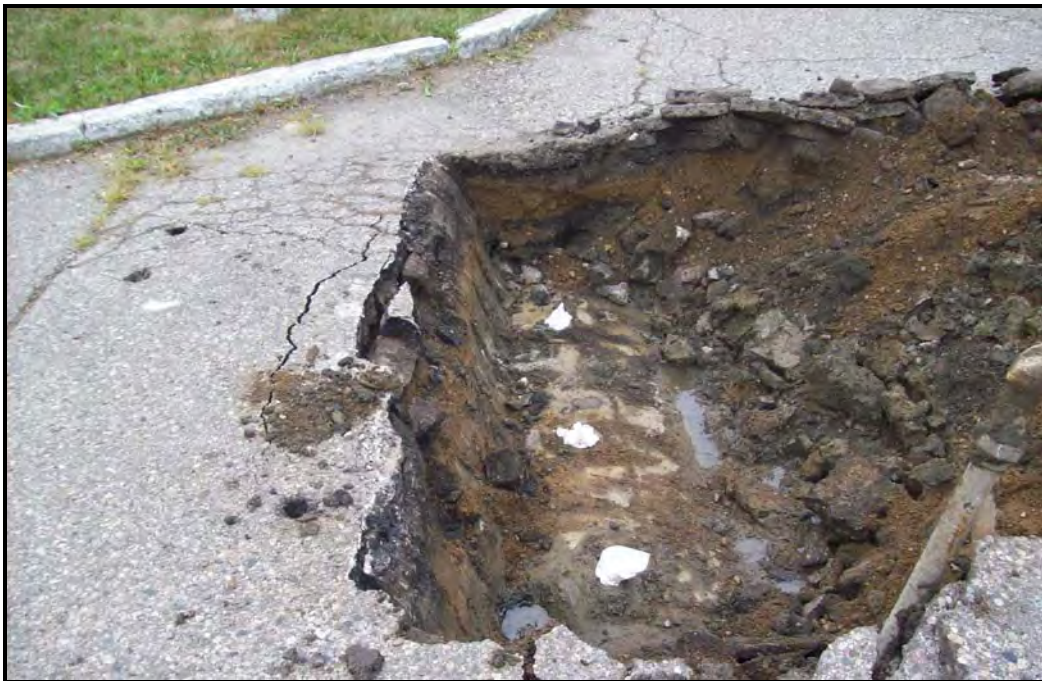
PHOTOGRAPH 6: 550-GALLON UST WITHIN TEST PIT #2
