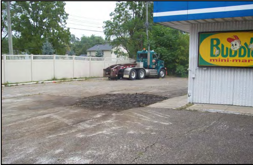
PHOTOGRAPH 9: TEST PIT #1 BACKFILLED
