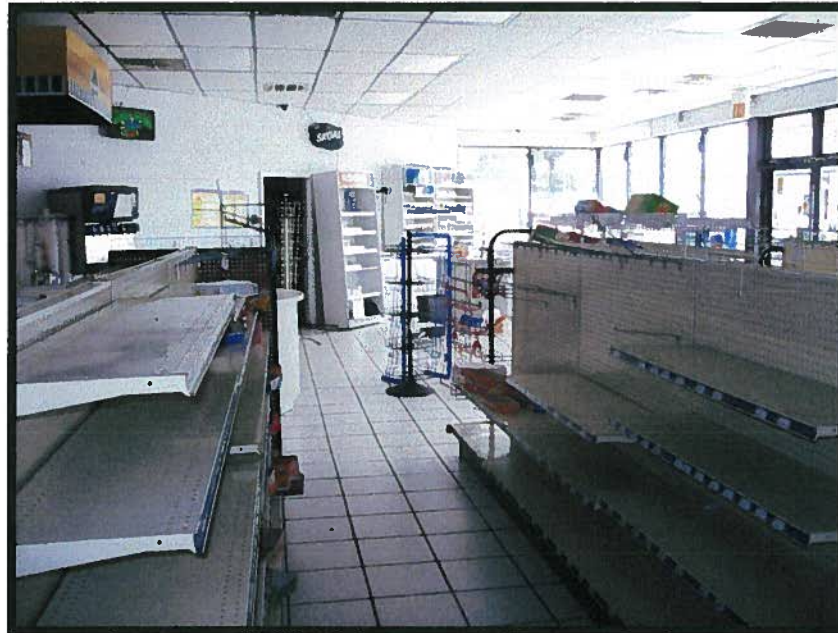
PHOTOGRAPH 4: SUBJECT PROPERTY GENERAL INTERIOR VIEW OF THE SUBJECT BUILDING
