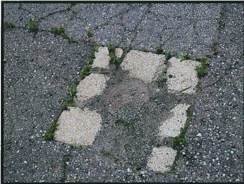
PHOTOGRAPH 8: SUBJECT PROPERTY VIEW OF A TYPICAL GROUNDWATER MONITORING WELL LOCATED THROUGHOUT THE SUBJECT PROPERTY
