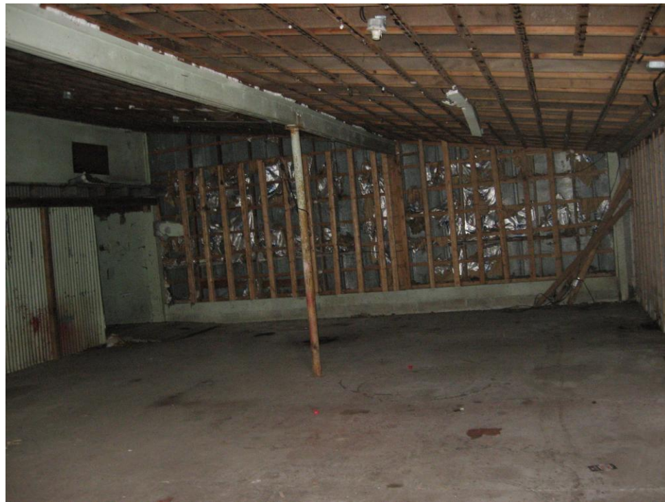
PHOTO NO. 10: North interior of storage building.
