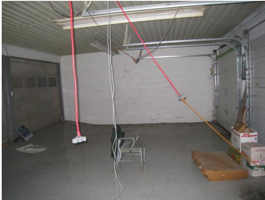
PHOTO NO. 5: Loading dock near southeast corner of manufacturing building.
