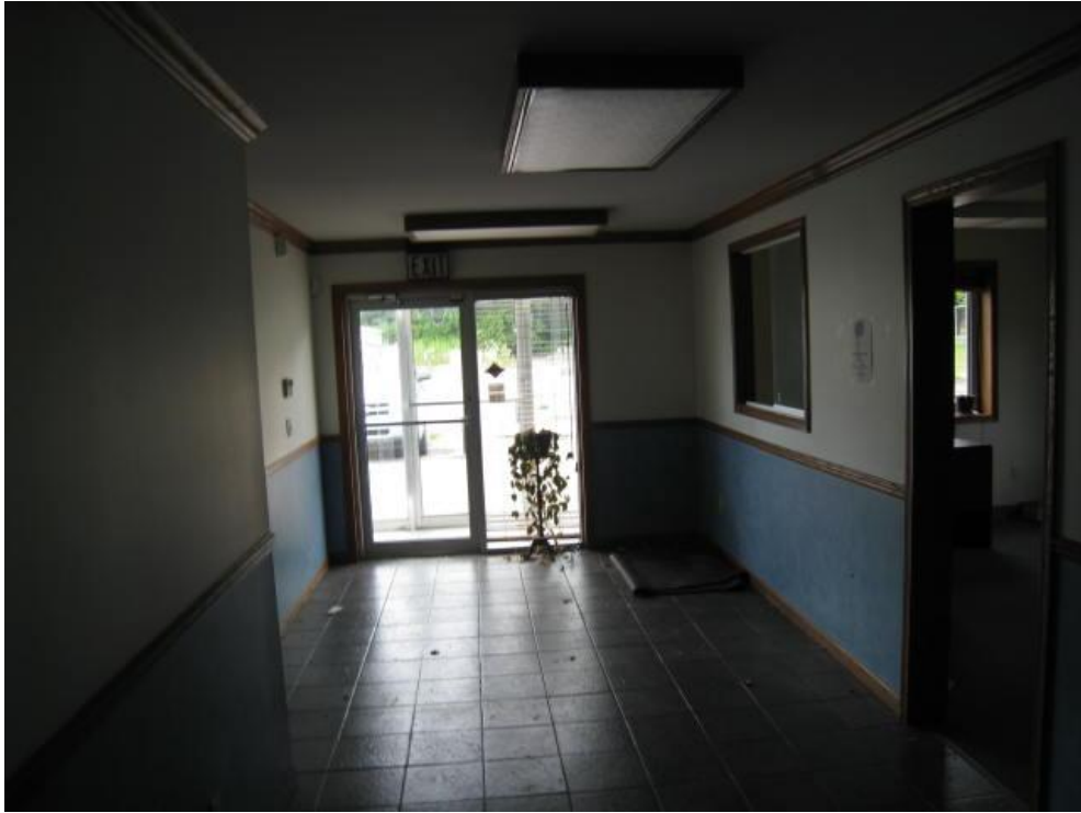
PHOTO NO. 1: Southeast entrance (office area) of the manufacturing building.
