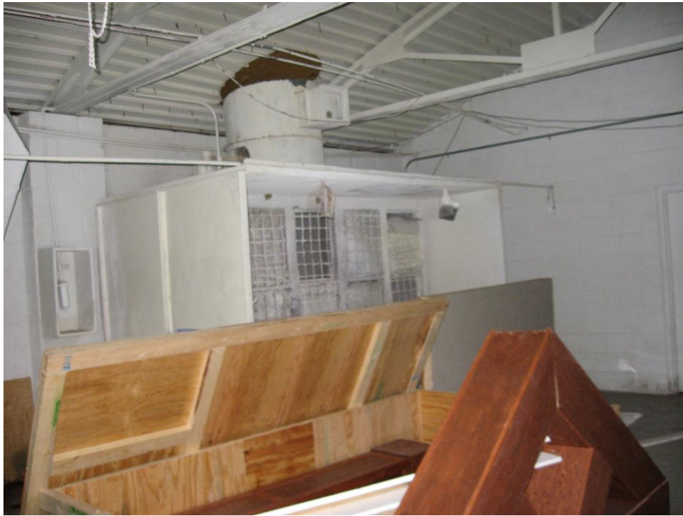
PHOTO NO. 7: Paint booth in manufacturing building.
