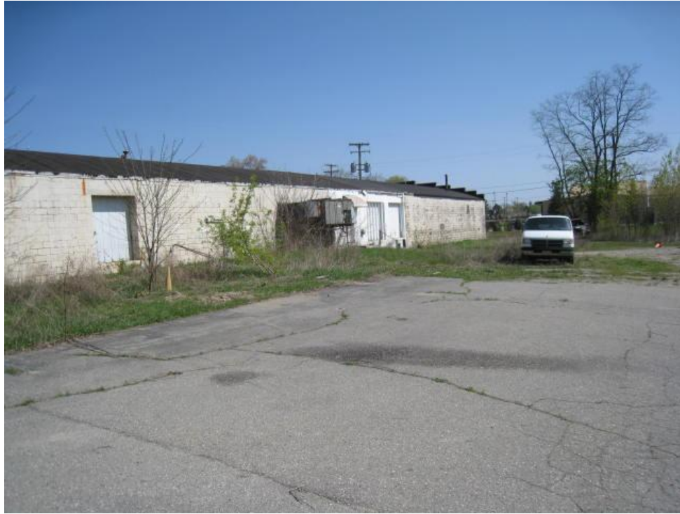
PHOTO NO. 3: Rear of the manufacturing building.
