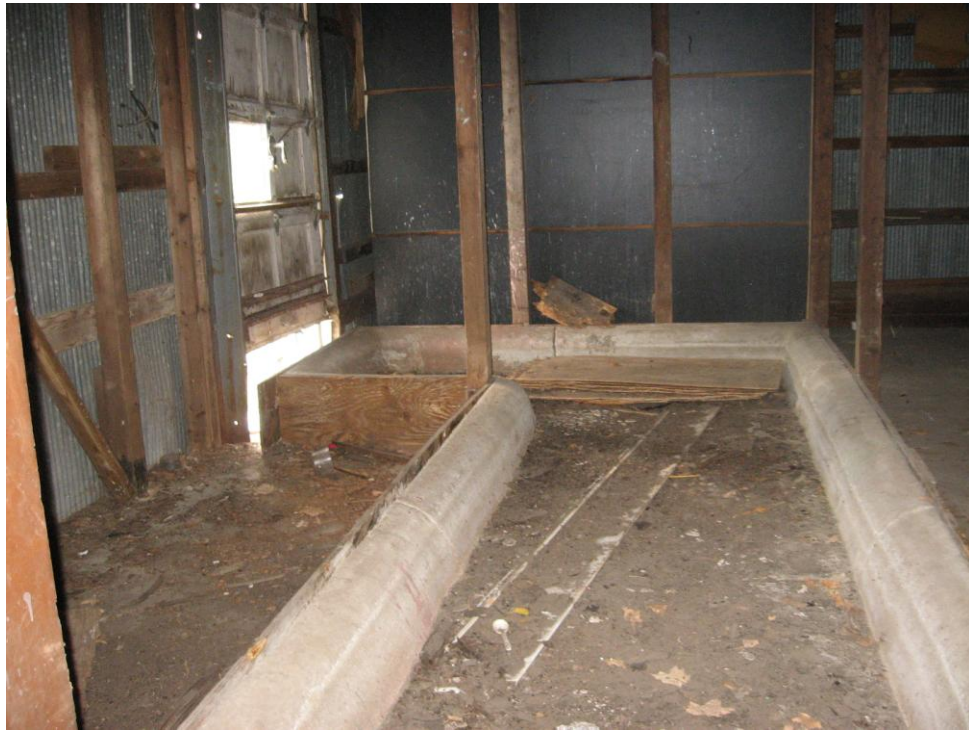
PHOTO NO. 11: East interior of storage building.
